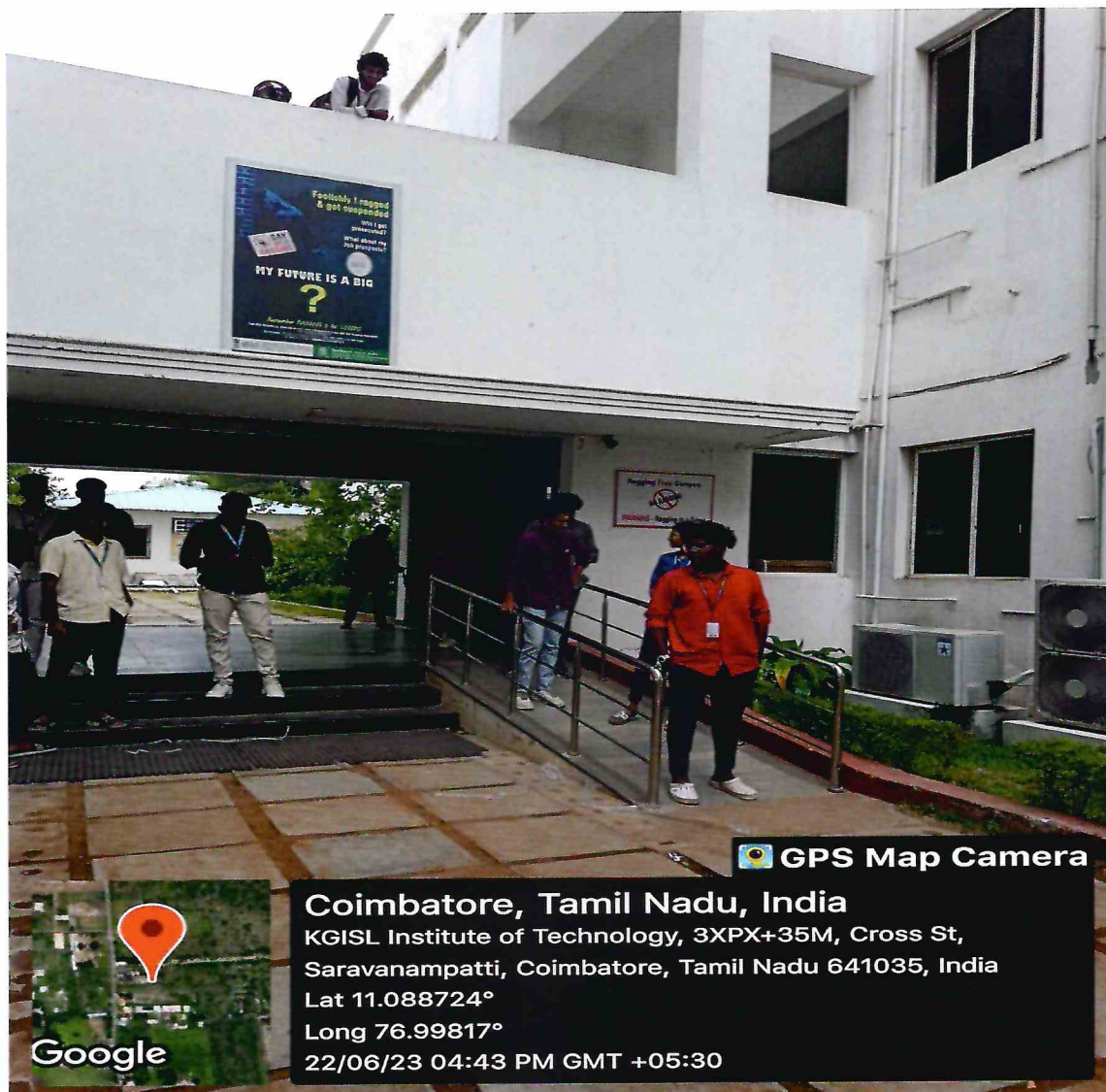
Ramp between academic and admin block
