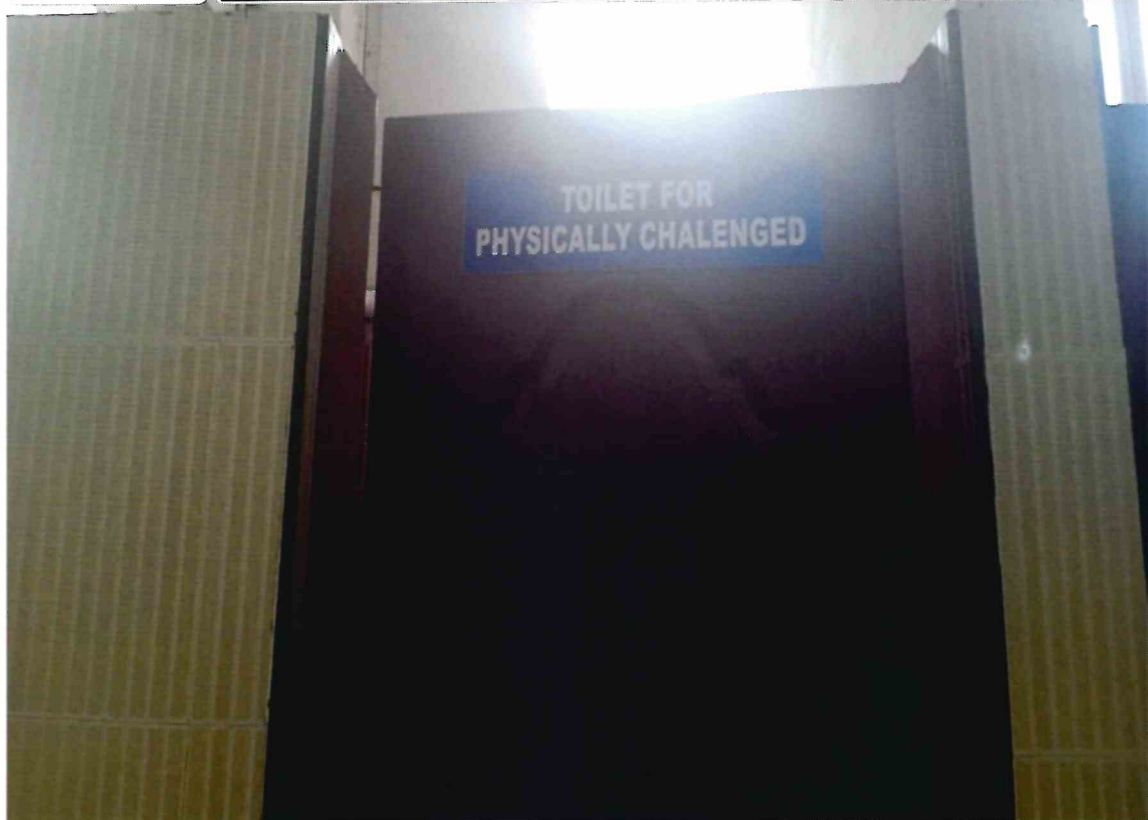
Sign Boards to differentiate the disabled friendly wash room with normal wash rooms
